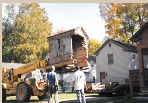
Being lowered onto a concrete slab
