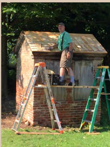
Vito laying shingles
