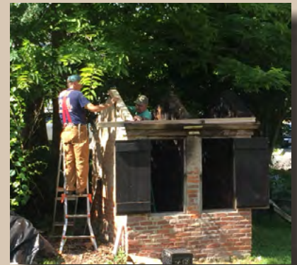
Paul O'Brien & Vito Valentini working on beams
