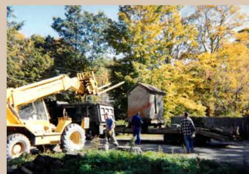
Forklift used to load onto truck
