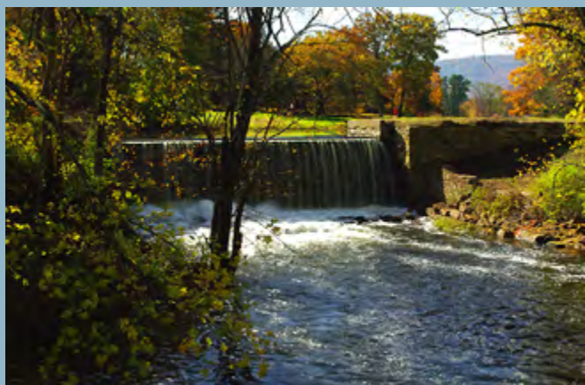
Spillway at Mill Pond
